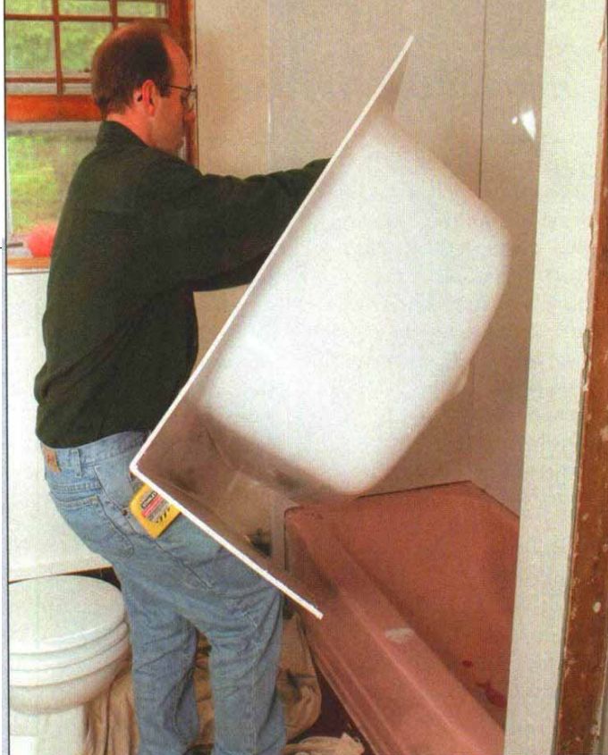
An old tub gets a face-lift. Chicago-based Luxury Bath Systems updates worn cast-iron bathtubs and aging tile walls with custom-molded acrylic replacements. No demolition is required.
